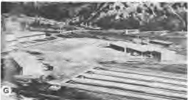
Fig. 29. FISH-REARING FACILITIES operated by the state today are primarily constructed with steel and concrete, and are equipped with sophisticated culture contrivances. The old frame-constructed hatcheries have all disappeared, or have been remodeled several times in the last 60 years.
