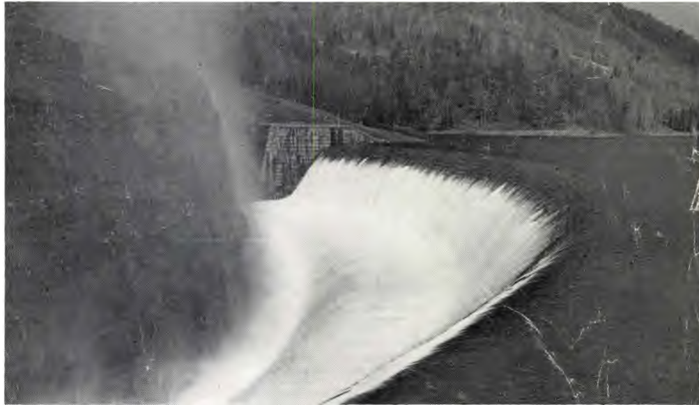
Pepacton Reservoir at spillway. More than 800 million gallons a day overflow when this photo was taken, April 18, 1956
